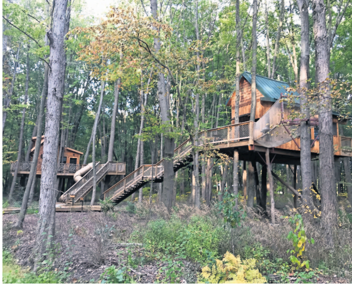
The Nest, left, and the Dragline, two overnight treehouses that are part of the new Cannalee Treehouse Village near Toledo.
