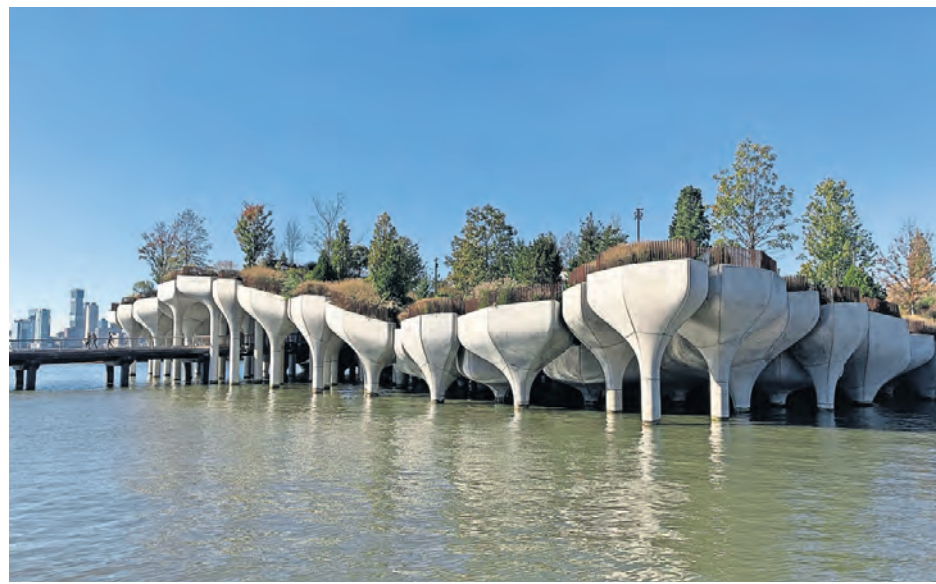
Little Island Park, built atop tulip-shaped concrete pilings in the Hudson River, is a new attraction in New York City's Meatpacking District.
