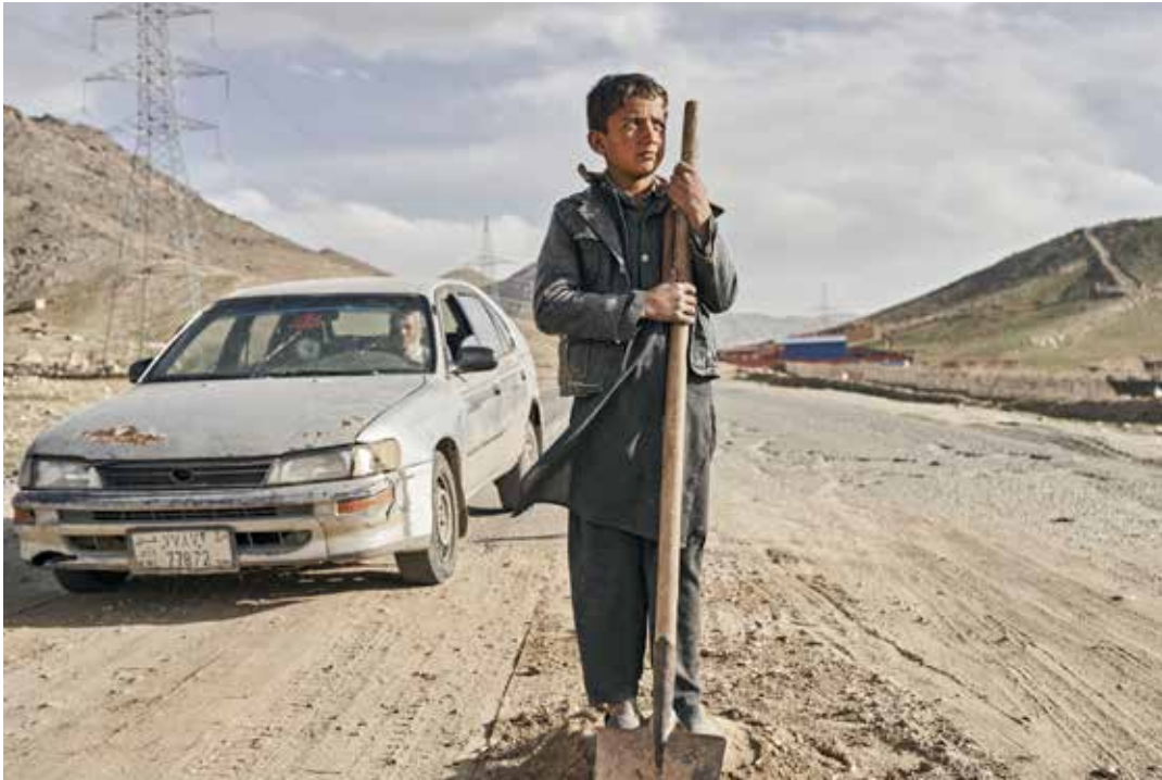
Rafiullah, 10, packs dirt into a bomb crater on Highway 1 near Maidan Shahr, Wardak Province. He and an older brother, like many boys who live near the Ring Road, serve as ad hoc repair crews, relying on tips from passing motorists to support their families.
